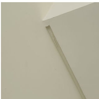
1. Painting of Walls and Ceilings
