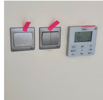
6. Electrical Switches & Sockets
